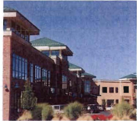
Required: Varied roof forms and depth help to reduce perceived building scale. False roof forms shall have depth behind the façade of the building no less than 25 % of the depth of the building footprint.
