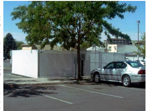
The privacy fence around the new compactor located at the Emporium Parking Lot 100 West 50 North in Logan.
