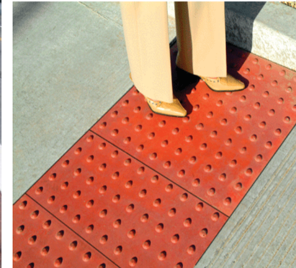
TRUNCATED DOMES - PRECAST CONCRETE TO MATCH BRICK
