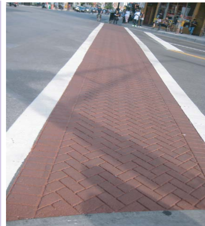
STAMPED ASPHALT CROSSWALK STANDARD DESIGN
