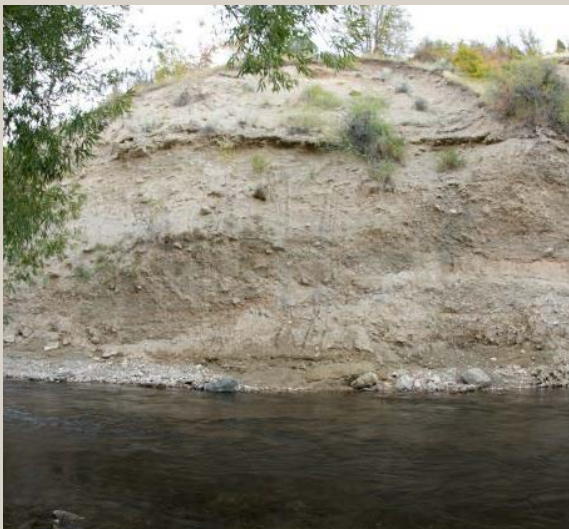
Example of erosion from the upper reach of the Logan River – erosion clogs the river with excess sediment.
