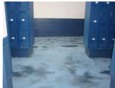
Logan Aquatic Center Skid Proof Flooring
